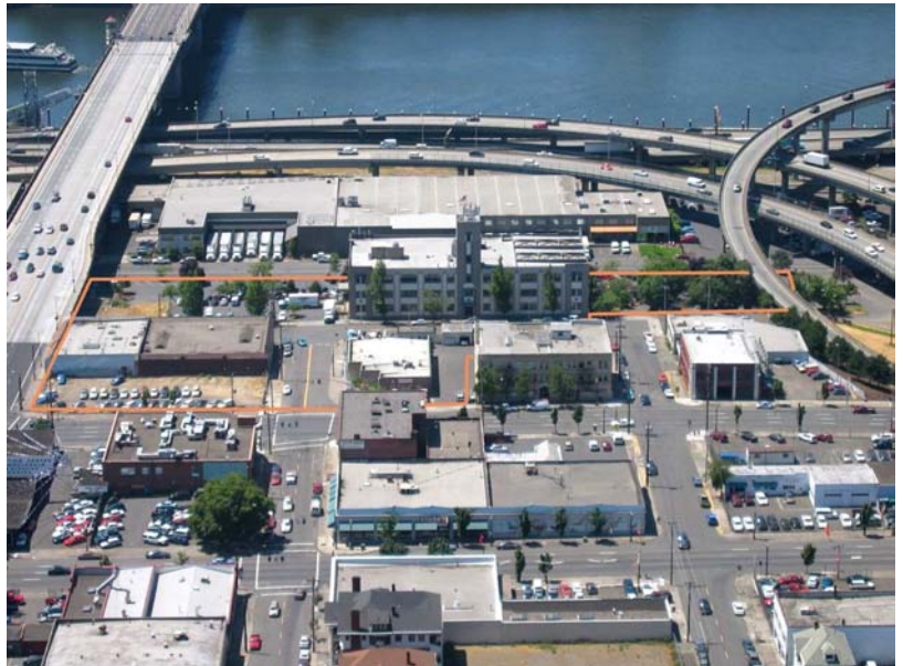
Burnside Bridgehead Site looking west.
