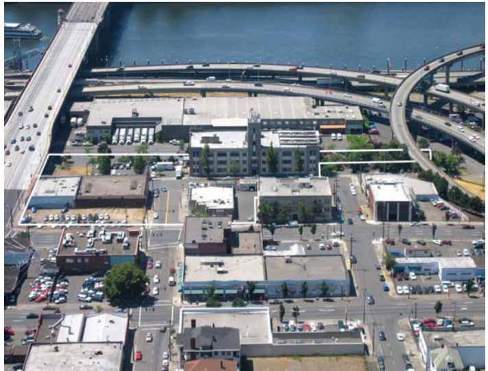
Burnside Bridgehead Site Looking West
