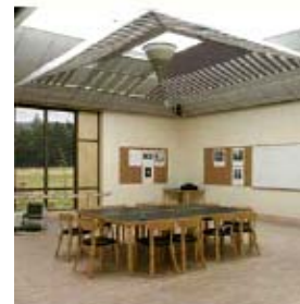
School in Mt. Angel, OR Photograph courtesy of Green Building Services
