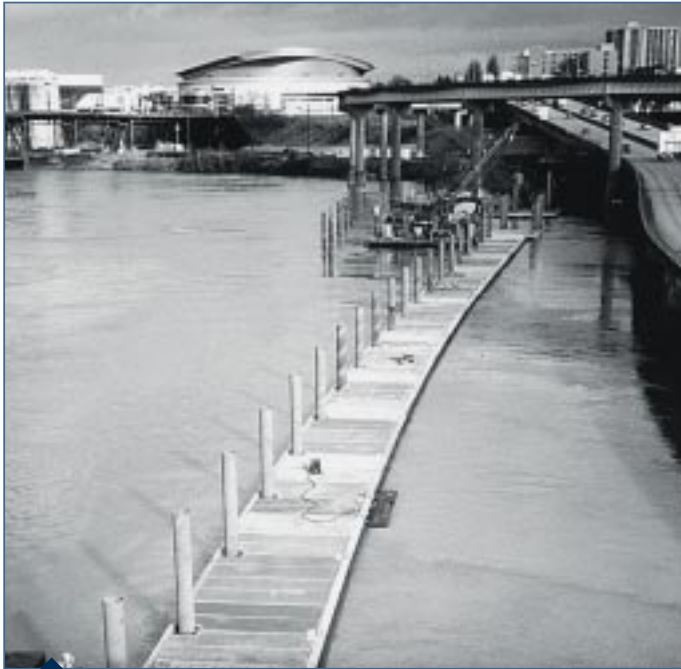
◆ The floating walkway begins to take shape at the Eastbank Riverfront.
